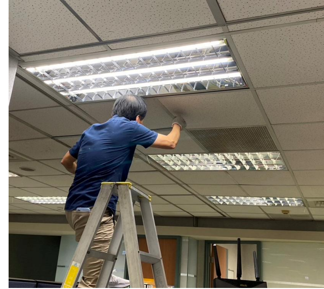
Replacing lighting sources with LED lamps
